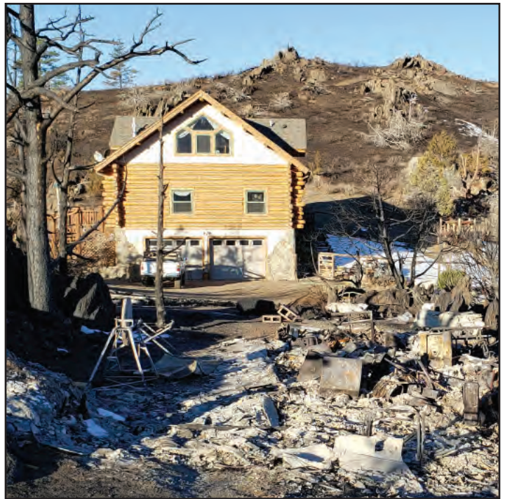
This log-cabin home survived the Cameron Peak Fire in 2020, but a workshop in the foreground did not. Photo by LaVonne Ewing.
