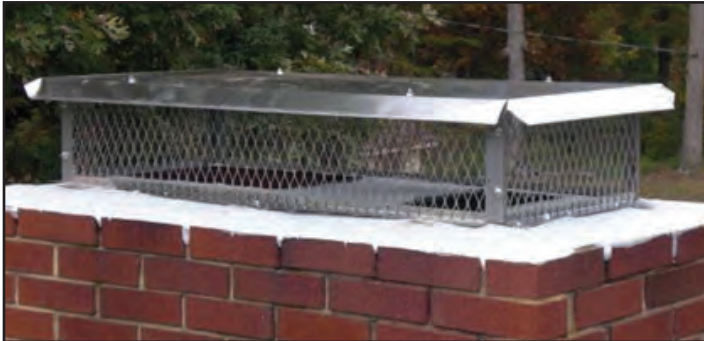
A spark arrester on a chimney. Photo by Colorado Springs Fire Department.
