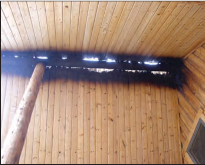
Damage to this wood home was limited to the ridge line, but screening the ridge vent could have prevented that damage. Photo courtesy of Rick Trenbath.
