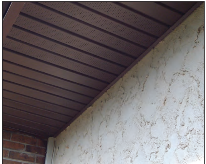
The eaves in the images above and below are protected by fire-resistant soffits. Photos by South Metro Fire Rescue.
