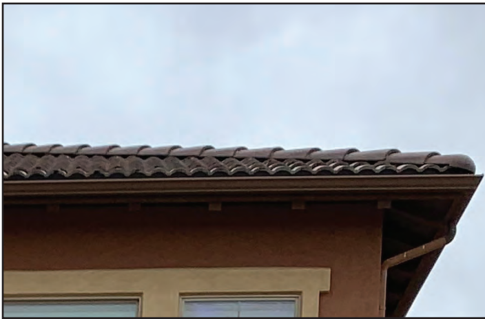
Although these roof tiles are curved, architects and builders were careful to form the layer below to prevent airborne embers from slipping under the tiles. Photo by South Metro Fire Rescue.
